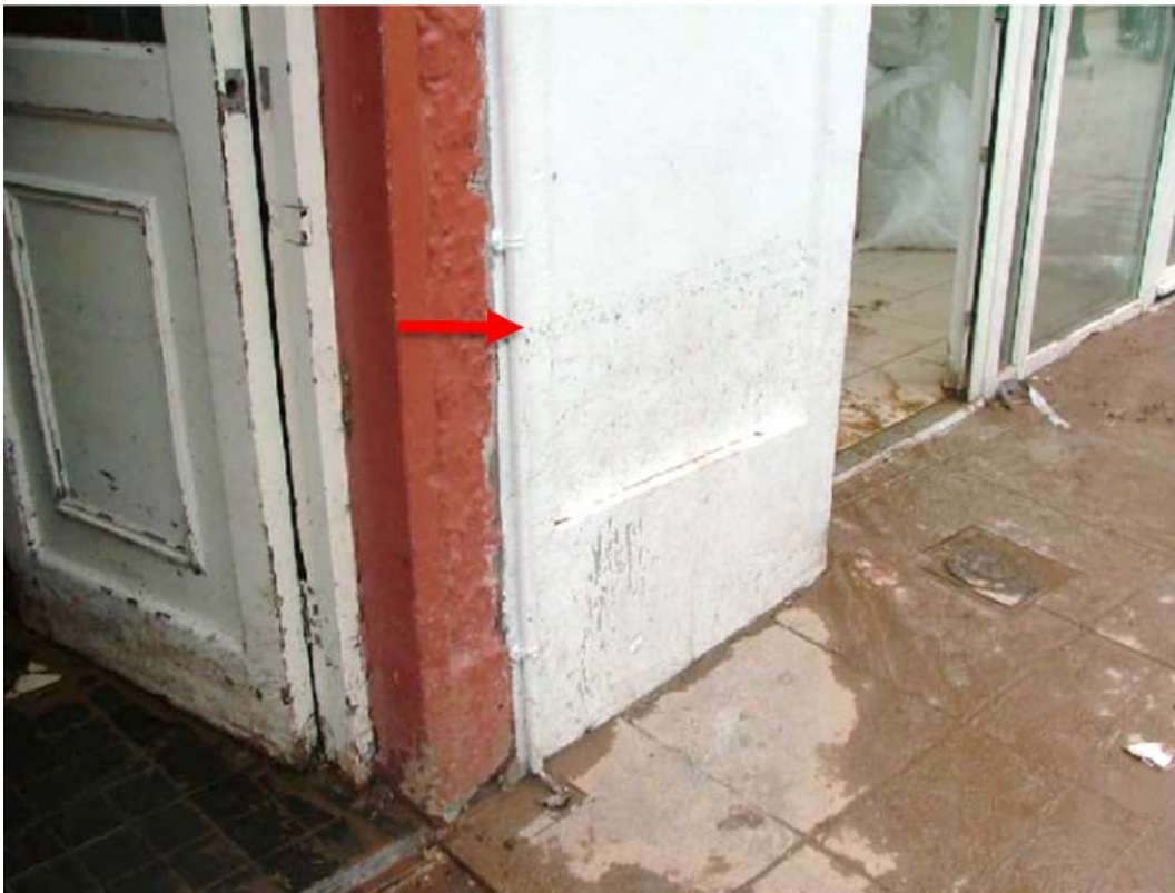
Figure 8.7: Post 2012 flood event high water mark from outside commercial property in Douglas East. Source: OPW
