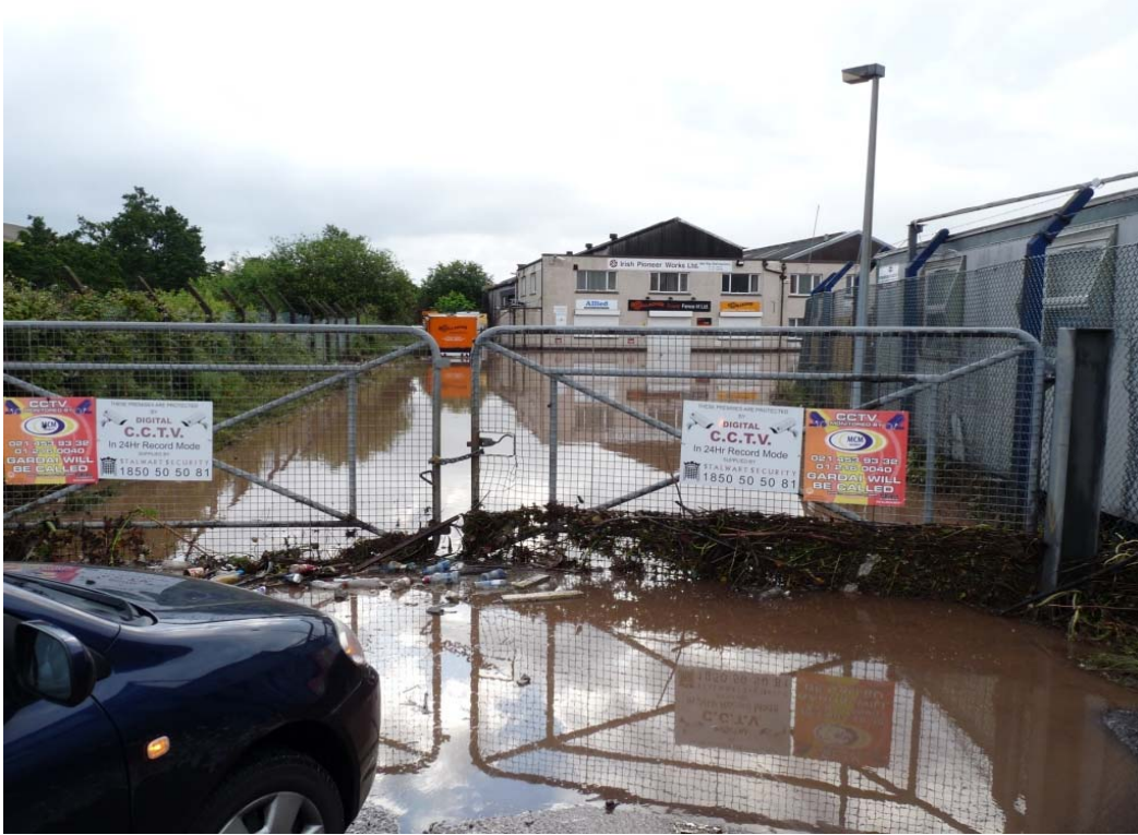
Figure 8.15: Post 2012 flood event in Togher Area. Source: Cork County Council
